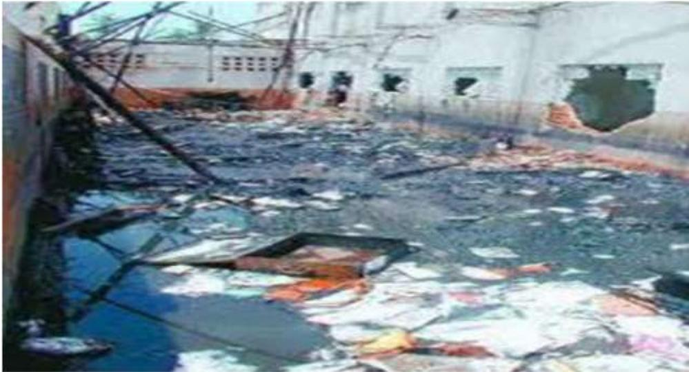
*This photo shows the top floor of the building. After consuming the fire the class room partition and the roof. Here there is no door, window, proper ventilation or escape route for each class room.*
